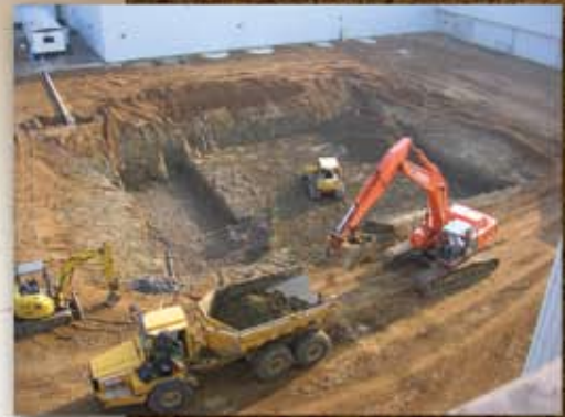
June 1 – Melt vault excavation began.
